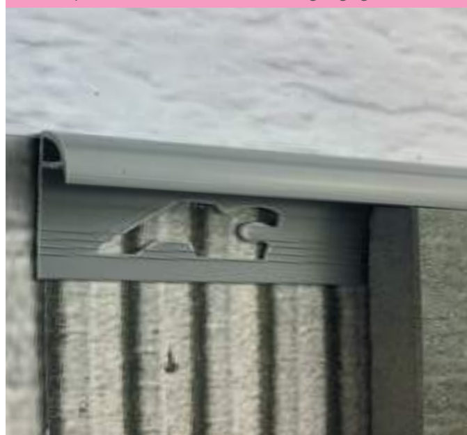
Chiusura perimetrale a muro/ Wall covering edging
