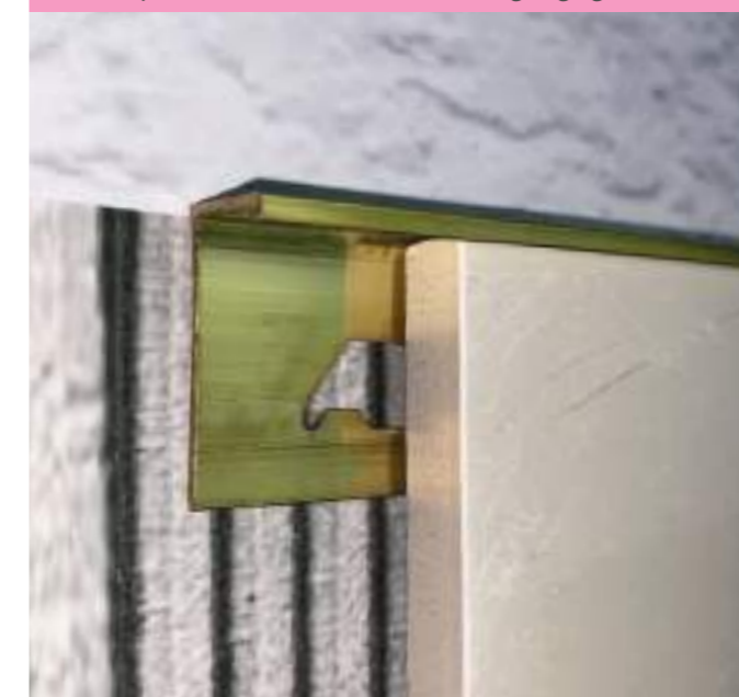
Chiusura perimetrale a muro/ Wall covering edging
