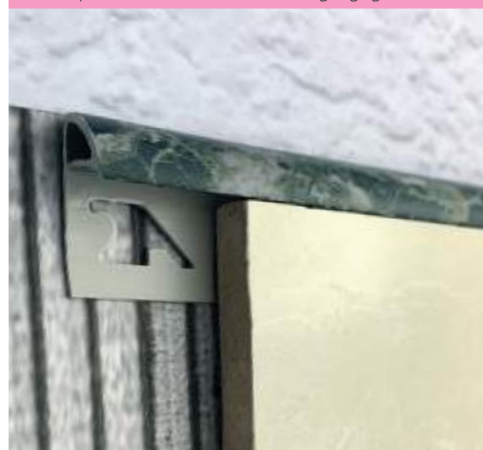
Chiusura perimetrale a muro/ Wall covering edging
