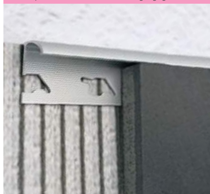
Chiusura perimetrale a muro/ Wall covering edging
